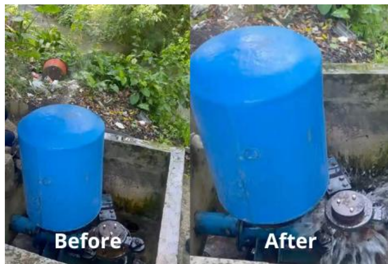
Figure 2. Condition of the pipes before and after hydam pump installation.
